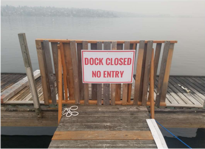
"Day dock" is permanently closed for safety
